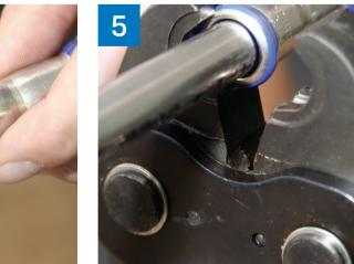
**Insert pipe into fitting**
