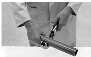
Cutting the pipe to length
