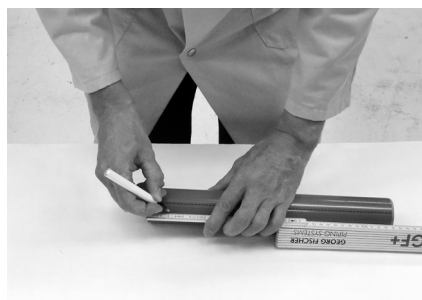
Marking the jointing length
