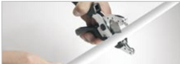
1. Cut pipe square and to length with pipe shears or pipe cutter.
