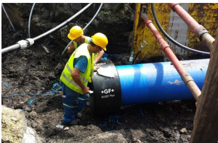
Picture 1: Installation of ELGEF couplers
