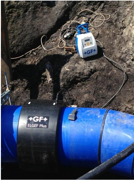
Picture 2: ELGEF coupler and MSA 2.1 welding machine
