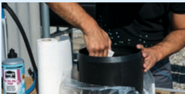
Clean the fusion zones of the fitting and pipe using a clean cloth.
