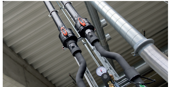
The ball valves type 546 in use in the printing house.
