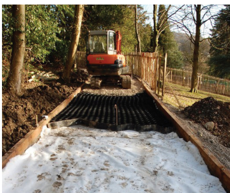
Fallbarrow Park, Windermere: CellWeb TRP® Installation
