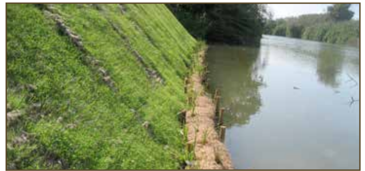
21.2 Embankment protection with GREENFIX products
