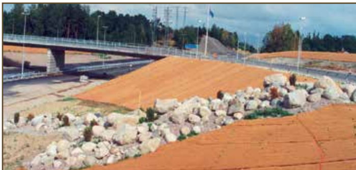
25.3 Mulchmat Installation in Sweden
