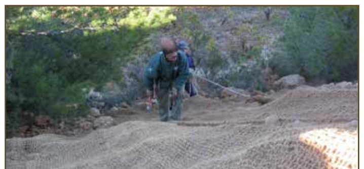
17.4 Installation of Greenfix Coir Netting KG0700 on a 50° slope
