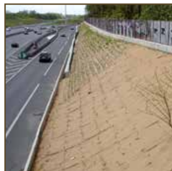
22.2 Mulchmat installation in south France
