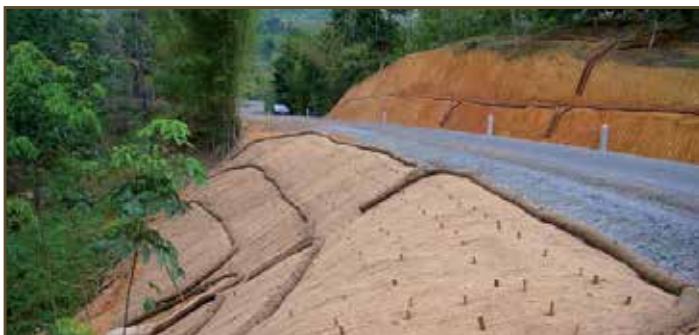
21.3 Slope application with Coir Logs
