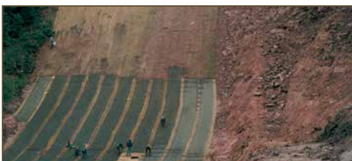
27.7 GREENFIX Covamat installation at a new Ski-Jump in RUHESTEIN
