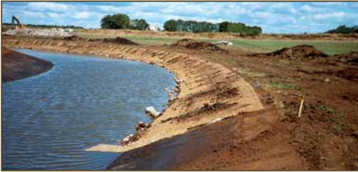
10.1 The use of Covamat plus with biodegradable nettings
