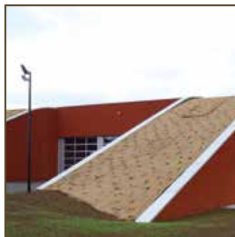
23.3 Creative roof-greening: Solution with Mulchmats never requires maintenance again
