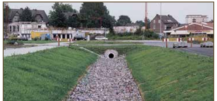
7.4 Strong root development and full vegetation establishment within 2-3 weeks after installation
