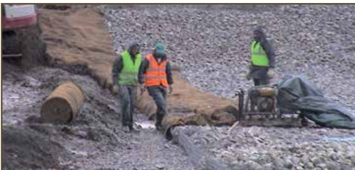
17.3 Shoreline Protection with Coir Netting KG0700
