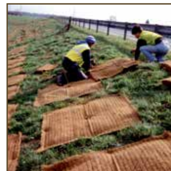
23.4 Norwich Bypass/ England: Individual plant protection with ready-slitted GREENFIX Mulchpats
