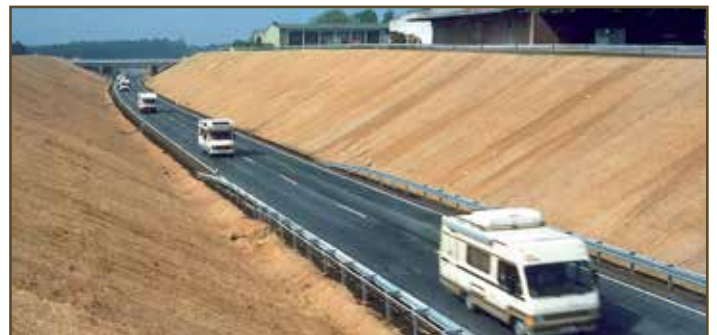
4.2 Slope was lightly seeded with customer's specific seed mix prior to blanket installation
