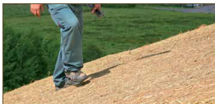
18.2 The easy and quick installation of GREENFIX Blankets
