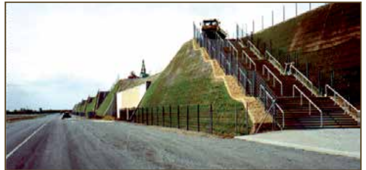
11.2 Vegetation of a retaining wall with GREENFIX f 3 blankets
