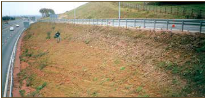
5.1 failed hydroseeded motorway slope
