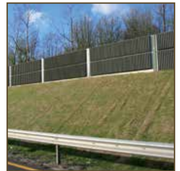
8.6 Immediate erosion protection with GREENFIX Eromat
