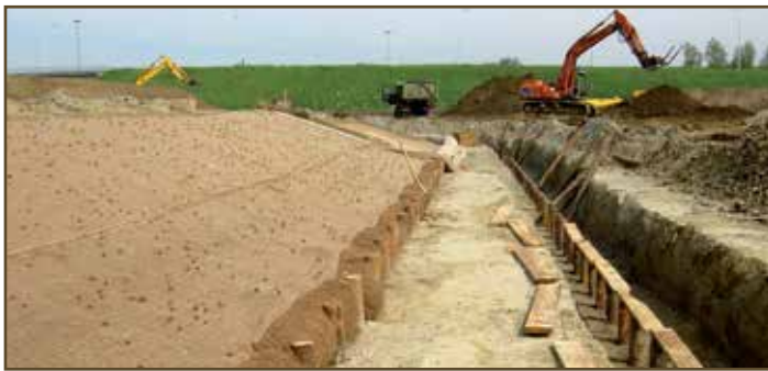
21.1 Channel application with our Coir-Logs
