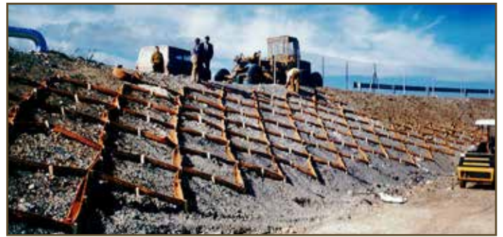
20.2 Filling the shapes with topsoil
