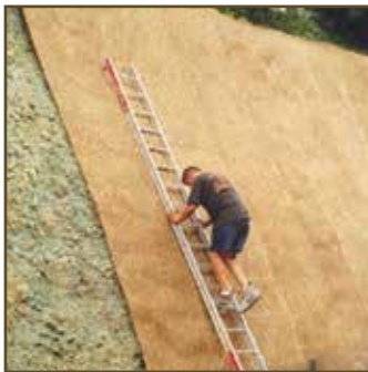
12.1 GREENFIX Rockmat Type 5D installation on 65° steep slope
