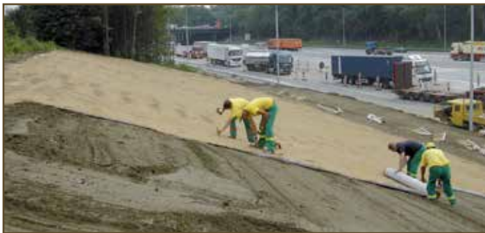
7.1 Approx. 60.000 sqm of GREENFIX Covamat fresh have been installed at the ring road of Antwerp/ Belgium
