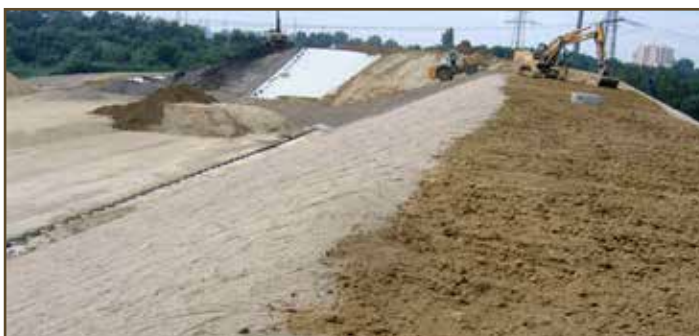
16.3 Installation on a 1:1,5 slope
