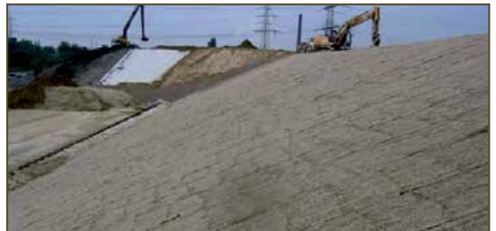
16.2 Immediate installation after end of construction
