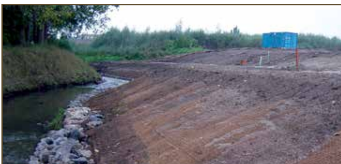
13.3 Ready installed Embankment Mat Type 700
