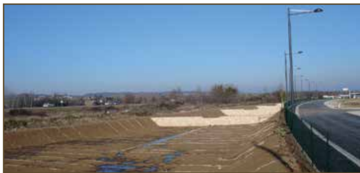
9.3 Application with GREENFIX Eromat Type 6B
