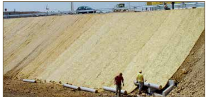
7.2 Motorway slope protection with GREENFIX Covamat plus in Lisbon/ Portugal
