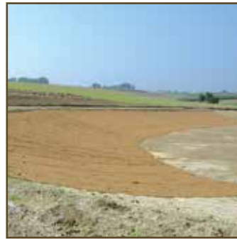
8.3 Application of GREENFIX Eromat for a retention reservoir (during installation)
