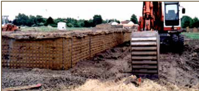
27.1 Gabion Construction at jobsite
