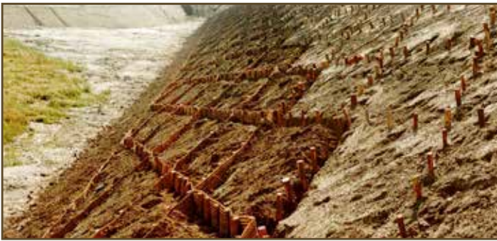
20.1 Recultex installation in diamond shape
