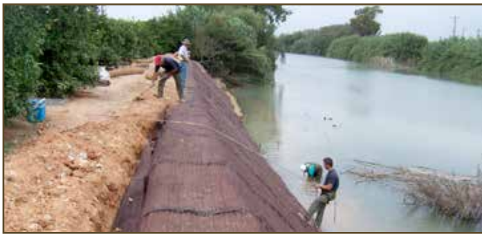
13.1 Shoreline protection with GREENFIX Type 75 C
