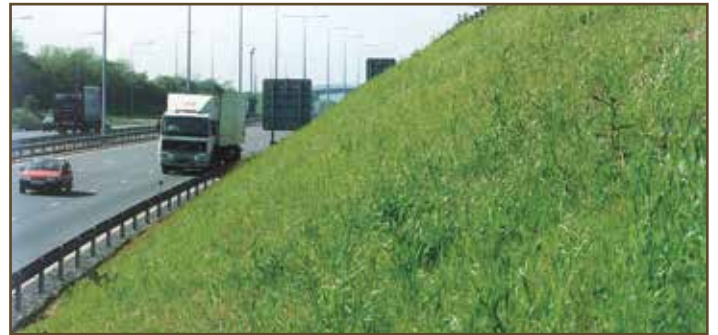
5.2 motorway slope prepared with Greenfix Covamat , vegetation established within 6 weeks
