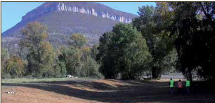
17.1 GREENFIX Coir Netting KG0900 in use on a tidal area of a river
