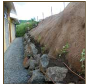
12.4 Successful installed GREENFIX Rockmat Type 6D in New Caledonia
