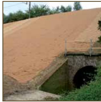
8.2 Slope protection with GREENFIX Eromat on a steep rail-road slope
