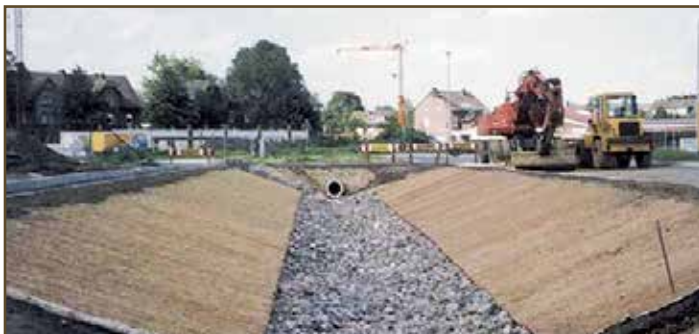
7.3 Protection of a road side channel with GREENFIX Covamat plus
