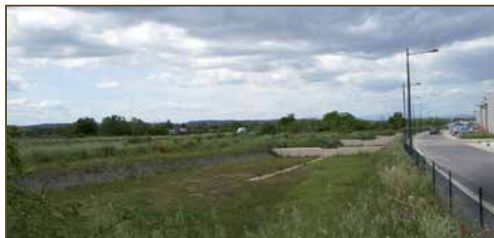
9.4 One year after installation
