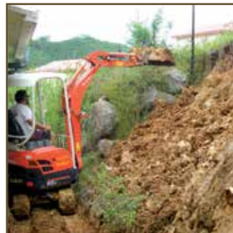
12.3 Preparation of a collapsed slope due to heavy rainfalls
