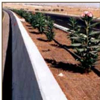
23.1 Highway on Cyprus: Economizing of irrigation water and less maintenance for reduced accident risk of workers
