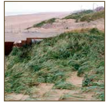
8.4 Marram grass transplants established through GREENFIX Eromat to stabilize dunes
