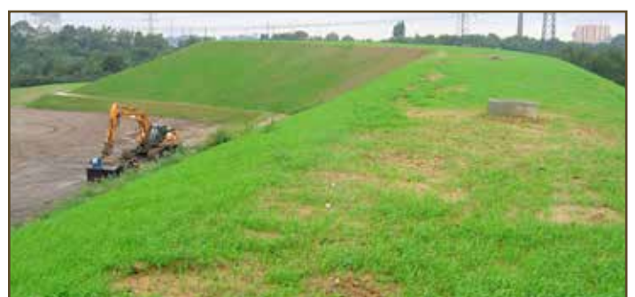
16.4 Five weeks after installation
