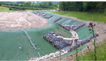
The completed PP5-Heavy Duty slope provides a secure surface once fully established and the permanent nature of the matting coupled with the Greenfix Anchor System ensures long term turf reinforcement and the immediate erosion control required by the constantly flowing water of the fish pass.
