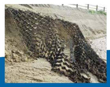
Substitute geocell project. Substitute geocells are often manufactured from inferior quality material that exhibits lower strength characteristics (i.e. seam strength). No project evaluation, no design collaboration and no contractor training or supervision can result in an improperly connected system in an improper application and with improper infill. Project Failure.
