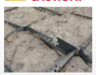
do not have the same material properties or design strength as the GEOWEB® material and can lead to a project failure.
