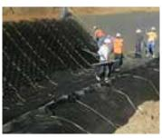
**CAUTION:** Other load transfer devices can become disengaged with the tendon and/or geocell cell wall, creating additional stresses that can lead to system failure.
