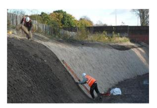
The benchmark low cost erosion control geotextile, GeoJute 500, has been specified for decades to provide cost affective protection to freshly cut or exposed slopes. GeoJute 500 offers a high degree of soil retention, before biodegrading completely to add to the organic content of the soil after sufficient time has passed for natural vegetation to establish and protect the soil from future erosion.
