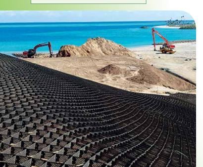
GEOWEB<sup>®</sup> slope protection systems may be designed with a variety of infill materials to meet project requirements for aesthetics, stability, environmental impact, material availability, and erosion-control. The system also provides protection to impervious liners.
