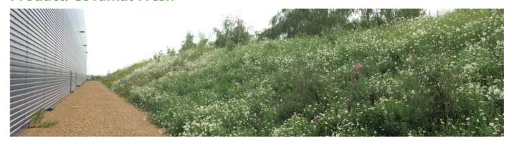
The project consisted of the installation of soil erosion protection and vegetation establishment to a newly formed slope at the recently extended DHL/Primark distribution centre at Thrapston near Kettering.
