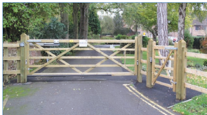
Uni-Gate at the school entry point
