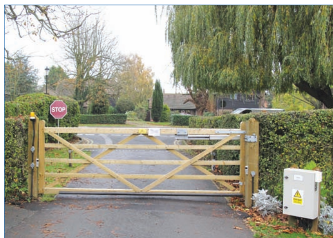
The 'exit' gate at the school with control box
