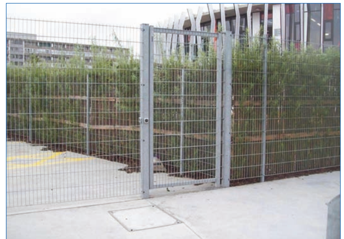
EuroGuard platform fencing and gate
