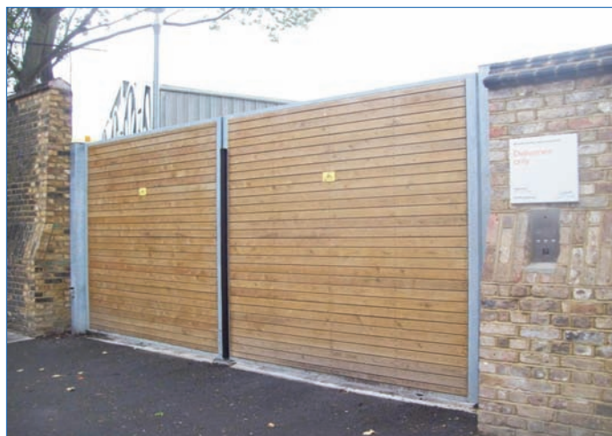
Steel framed automated gate with tongue and groove cladding
