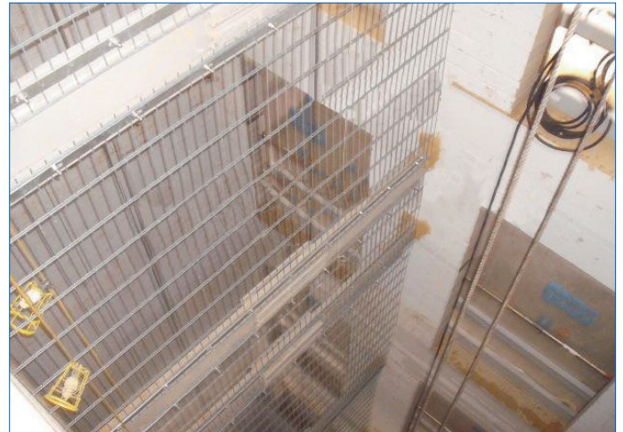
60m lift shaft clad with EuroGuard
