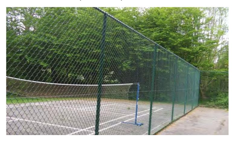
Our tennis court system is made from Tubular System 3. Single courts are 18m x 36m with one gate, and double courts are 34m x 36m with two gates. Posts can be supplied in either a galvanised or powder coated finish in our standard colours.
