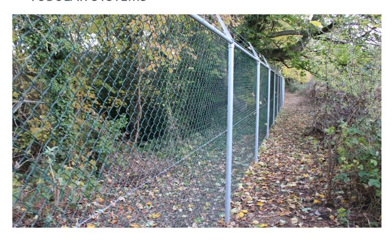
Unlike generic systems, Jacksons Tubular Systems for Chain Link and Welded Mesh fencing can feature a top rail for added security and strength. They are made entirely from steel, galvanised as standard or galvanised and powder coated to BS EN 13438 in one of our standard colours.
