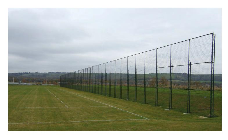
Jacksons was the first to develop the double lattice post design for our Ball Stop Fencing in 1994, which provided a structure strong enough to allow sports webbing / mesh to remain in place safely throughout the year. While many have imitated the design, none have bettered it. That's because we prioritise use of the best materials in our proven design, including our top rail for extra rigidity to ensure durability and safety for both users and the public.
