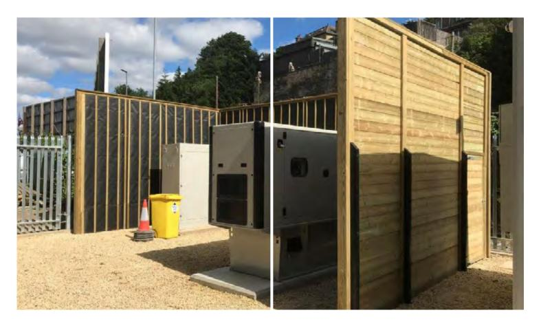
\*Jakoustic® barrier certified laboratory results: Rating according to BS EN 1793- 2:1998; Category = B3. Rating according to BS EN 1793-1:1998; Category=A3. Laboratory sound reduction 32dB.
