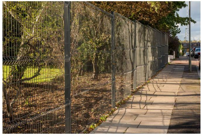
Euroguard<sup>®</sup> Regular is ideal for residential areas, commercial properties, schools or car parks. The "V" shaped profile reinforcing folds increase the panels rigidity and strength. Panels can be stacked above one another to deliver a higher fence.
