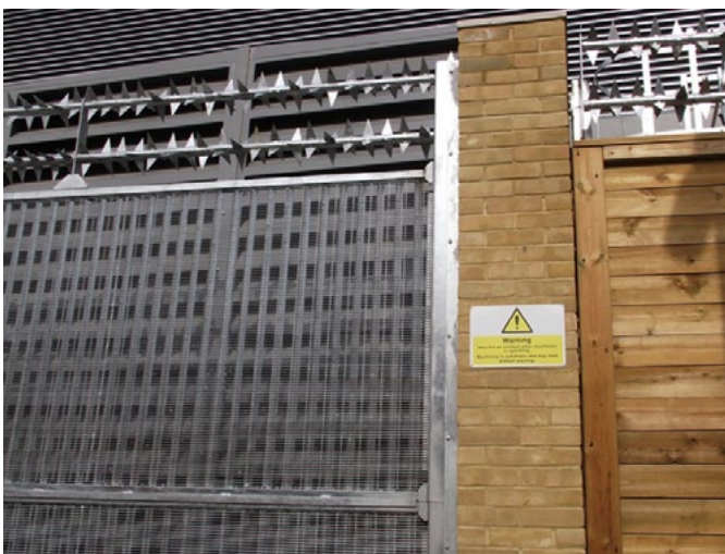
Trident Xtreme 3 System Gate with Rota Spike Topping
