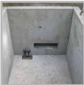
Once-piece chamber with inlet and outlet holes
