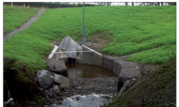
Complete landscaped Hydro-Brake® Installation.
