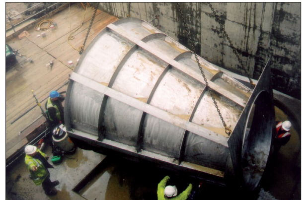
Installation of the Hydro-Brake® Flow Control at Weedon Dam.
