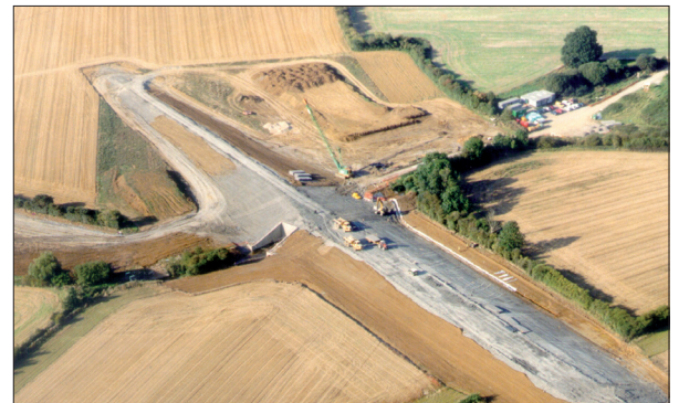
Aerial view of the dam during construction.
