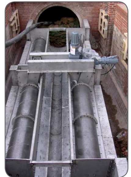
Carlisle Street Heliscreen® installed in the chamber.
