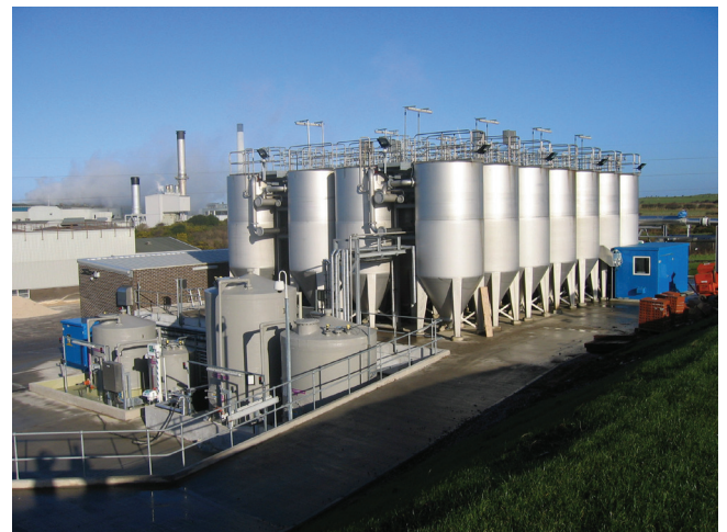
Installed DynaSand® Filters and Lamella® Plate Clarifier
