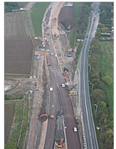
Project under construction
