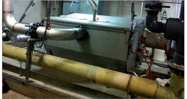
Hydro MicroScreen™ - a small footprint replacement for primary clarifiers
