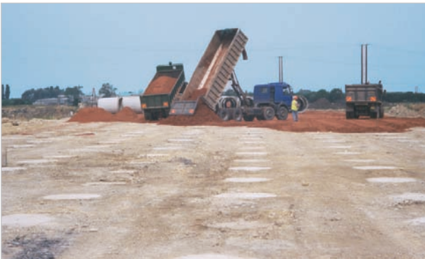
Picture 3: Preparing the regulating layer over pile heads
