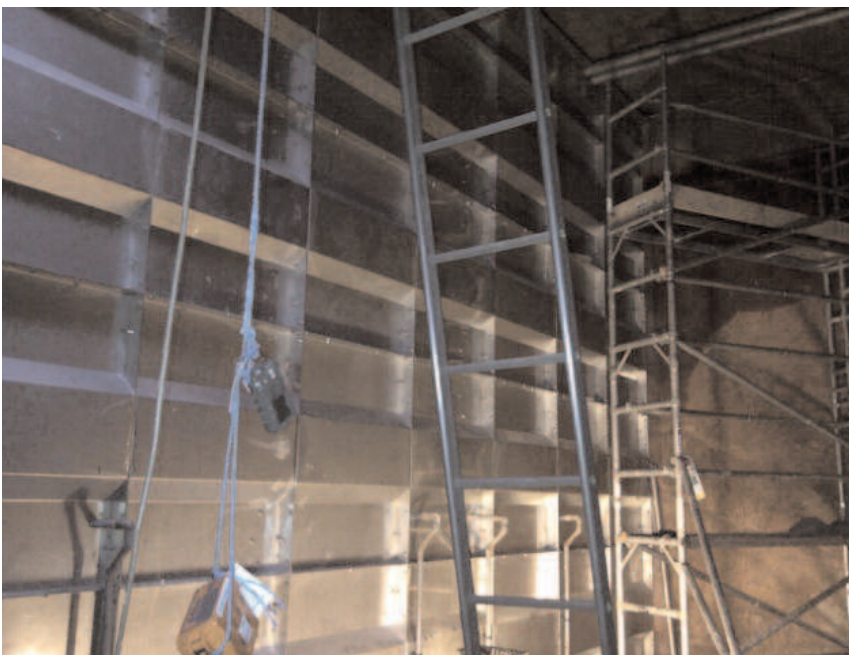
Walls nearing completion
