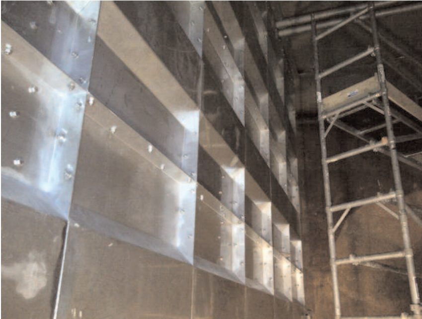
Close up of installed panels
