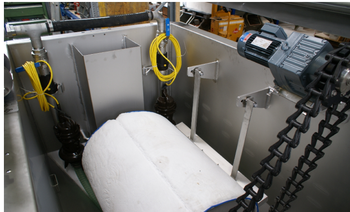
Pile Cloth Media Filter in a drum configuration at Willand WwTW
