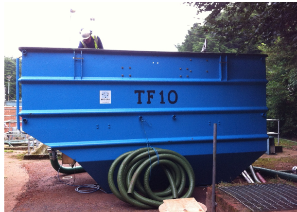
TF10 (Willand WwTW)
