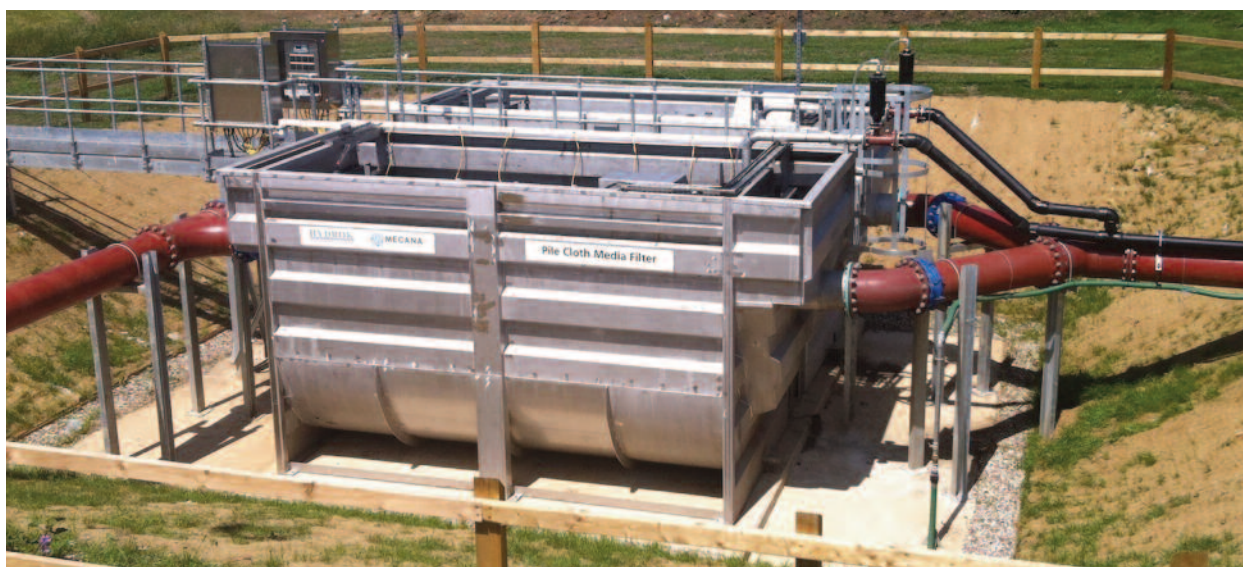
Figure 1 & 2: Installed SF15/75 Mecana Pile Cloth Filter including access metalwork
