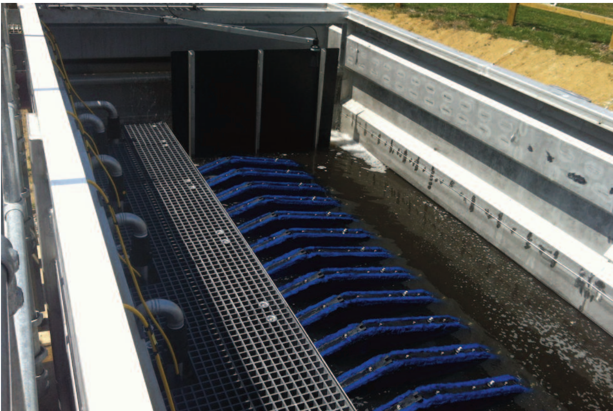
Figure 4: Installed SF15/75 Mecana Microfibre Cloth Filter including access metalwork
