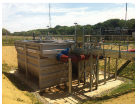
Figure 1 & 2: Installed SF15/75 Mecana Pile Cloth Filter including access metalwork
