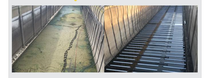
Planned cleaning helps to extend the life of PCMF material and aeration diffusers
