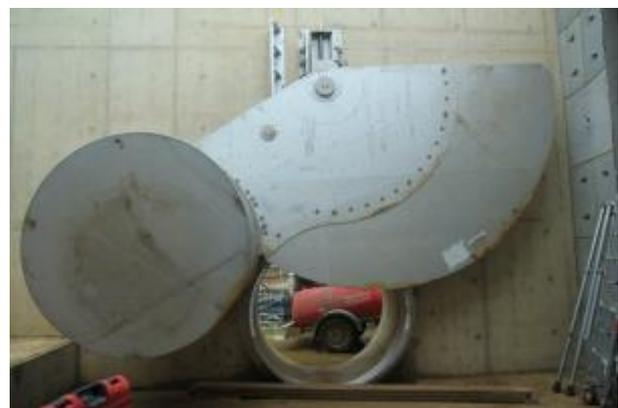
Accepting some moving parts, and therefore maintenance, allowed the HyrdoSlide to be considered. A HydroSlide consists of see-saw on a pivot with a plate at one end and a float as the counter balance at the other. As the water level increases the float rises causing the plate to close across the orifice opening and restricting outflow. Although it has a moving part, the discharge curve holds tightly to the optimum discharge, plus or minus five percent.
