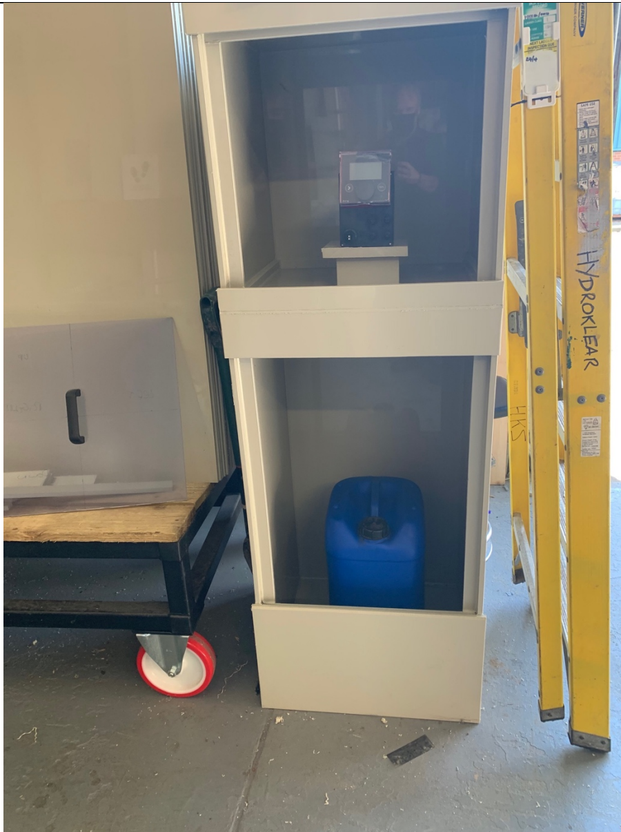
Single pump c/w small bund – Local pipe work etc. to be added in
