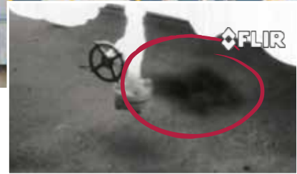
Captured gas leak from production site.
