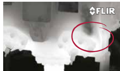
Captured gas leak.
