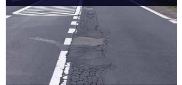
Fatigue cracking
