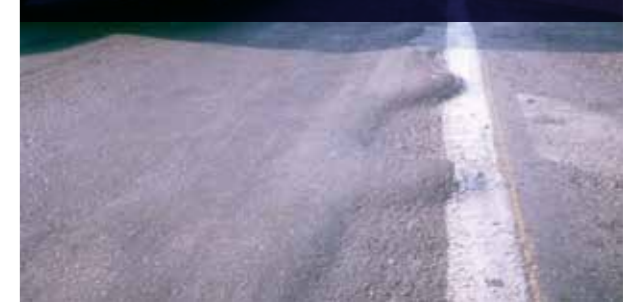
Rutting and shoving
