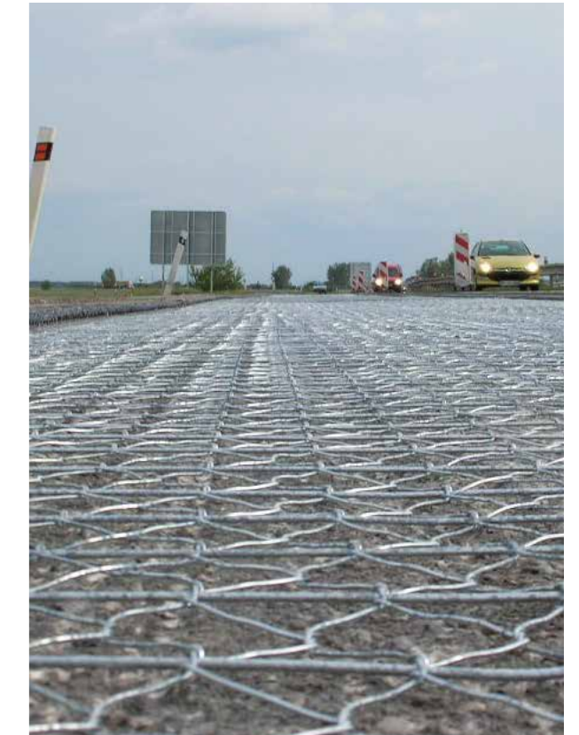
Road Mesh® provides lateral restraint to the asphalt which improves resistance to rutting and shoving
