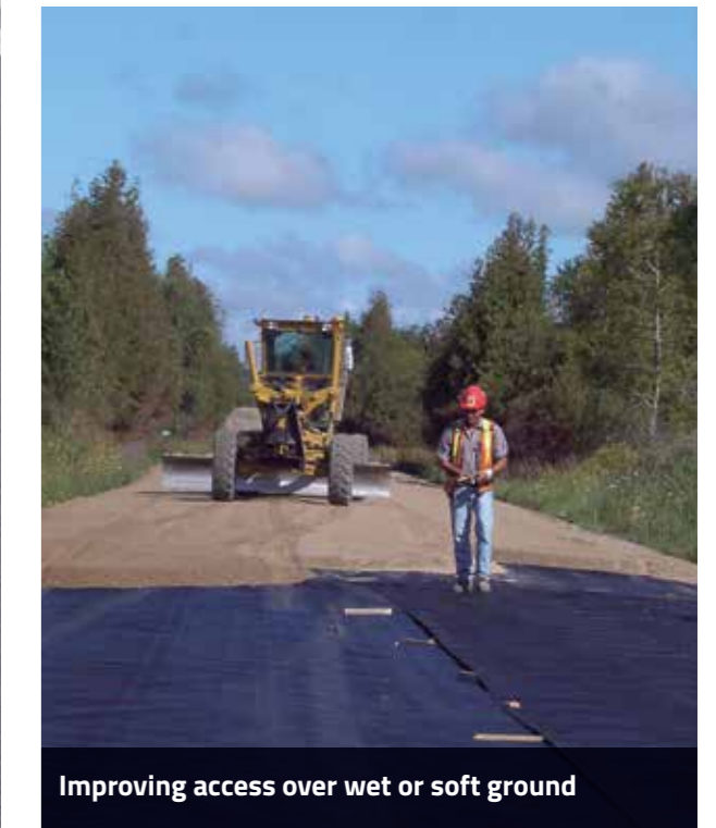
Reinforcing pavements over peat
