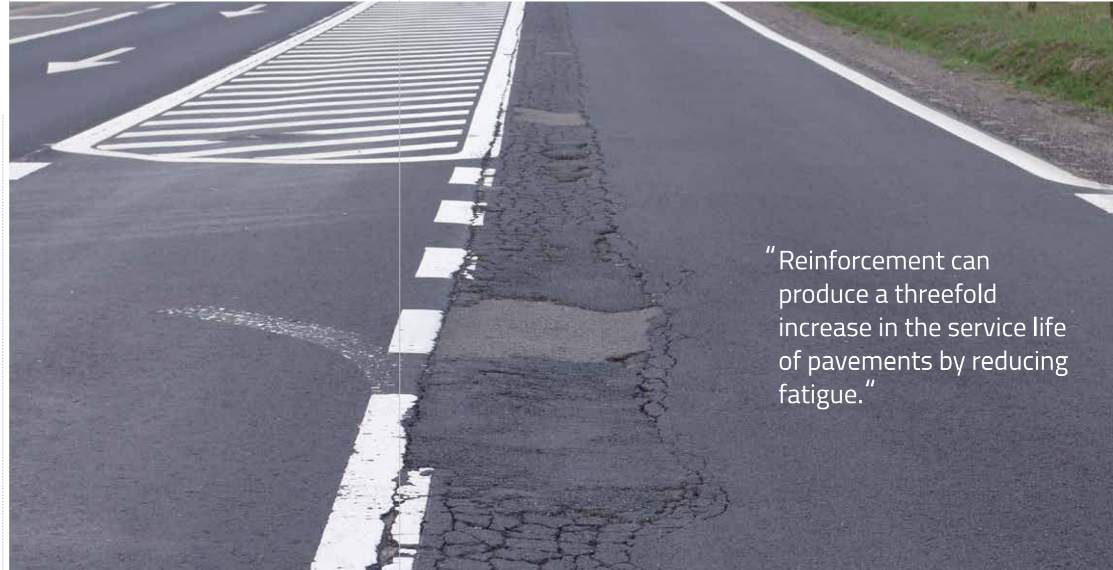
Reinforcing pavements over peat
