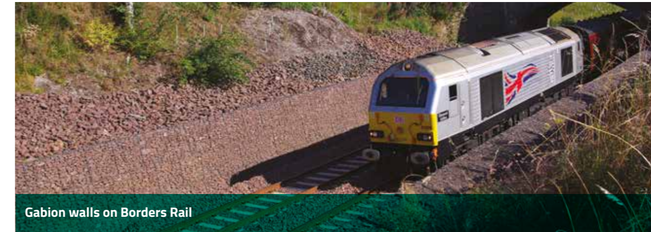
Green Terramesh® supporting a railway line
