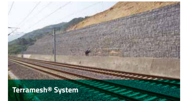
Green Terramesh® supporting a railway line
