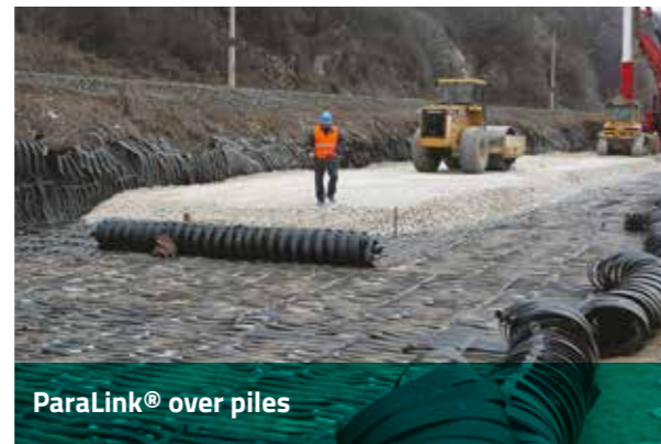
ParaLink® basal reinforcement over soft soil
