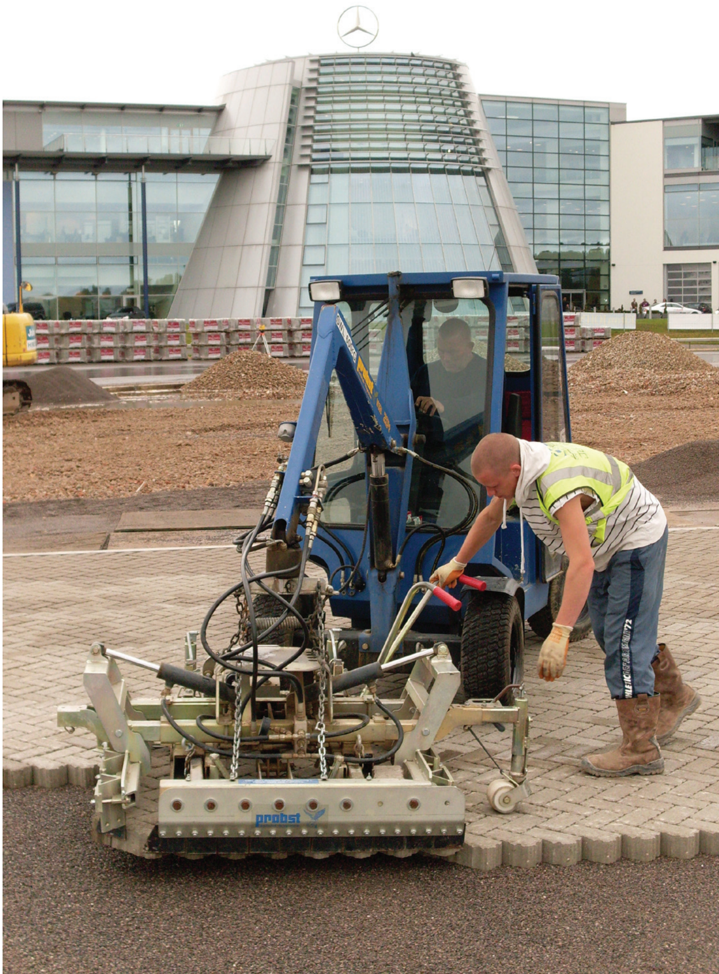
Installation in progress
