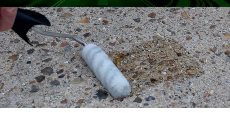
Spectrum UltraPrime is a methacrylate (MMA) primer. Used as a primer for concrete and cementitous surfaces, prior to the application of Spectrum UltraGrip, UltrStripe, and Ultraforce MMA coating systems.
