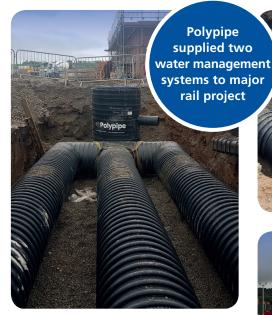
RIDGISTORMSeparate Catchpits were installed to separate the water from other particles with petrol interceptors to ensure safe and clean discharges into the local water networks. The water is dispersed from the attenuation tanks through a system of RIDGISTORMCheck chambers, which controls water discharge at precise rates using penstocks and vortex flow controllers.
