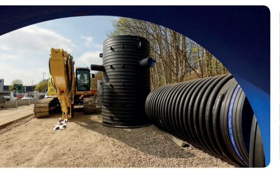
Polypipe Ridgistorm-XL large diameter pipe and chambers have been installed beneath a live carriageway, in an innovative design solution that saves space while providing the required surface water storage for a highway upgrade.
