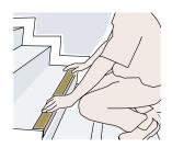
When on-site, check step measurements with cut Stair Nosing supplied. Trim if required. Prepare step edge surfaces. They must be clean, smooth and clear of debris.
