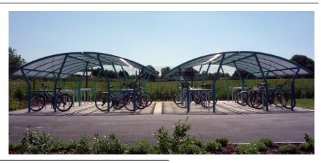
The Canterbury Cycle Shelter is an extremely robust and classically designed, free-standing cycle shelter designedfor on site assembly, constructed from galvanised steel and PET sheet. The VELOPA Canterbury Cycle Shelter is a popular design that exemplifies the AUTOPA approach to cycle parking, the shelter is designed and fabricated to look good for years. The frame is made from 76mm galvanised mild steel round tube. The roof is available in either polycarbonate or corrugated steel.
