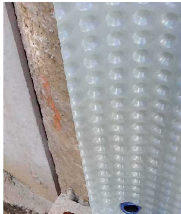
Cavity Drain R7 In Situ
