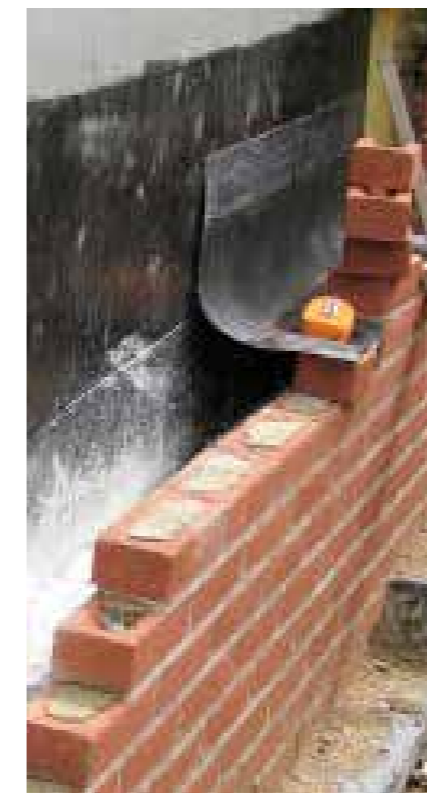
Typical Cavity Tray In Situ
