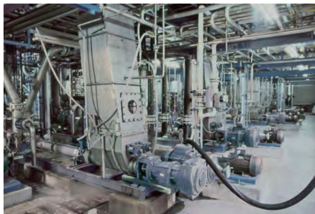
Pumps of range BTI 35-24 Conveying products: Sulphite- or sulphate stock Conveying capacity: 2.8 – 20 m 3 /h (12 – 88 GPM) Pressure: 16 bar (232 PSI) • Temperature: 20 – 90 °C (68 – 194 °F)
