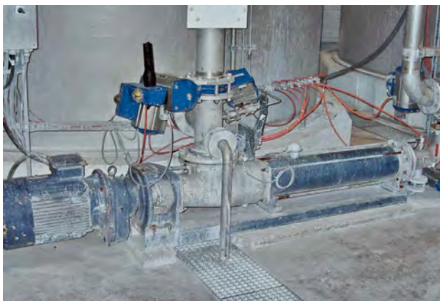
Pump of range BN 130-6L Conveying products: Coating and glue Conveying capacity: 40 m 3 /h (176 GPM) • Pressure: 4 bar (58 PSI) Temperature: 24 – 50 °C (75 – 122 °F)
