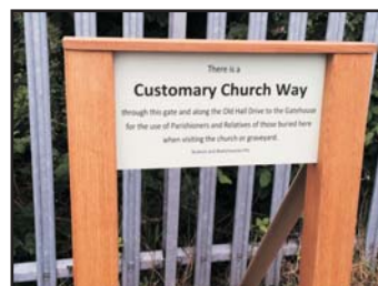
F10. Side mounted posts and weather board.
