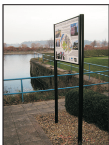
V5. Side mounted posts.
