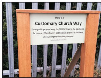
F10. Side mounted posts and weather board.
