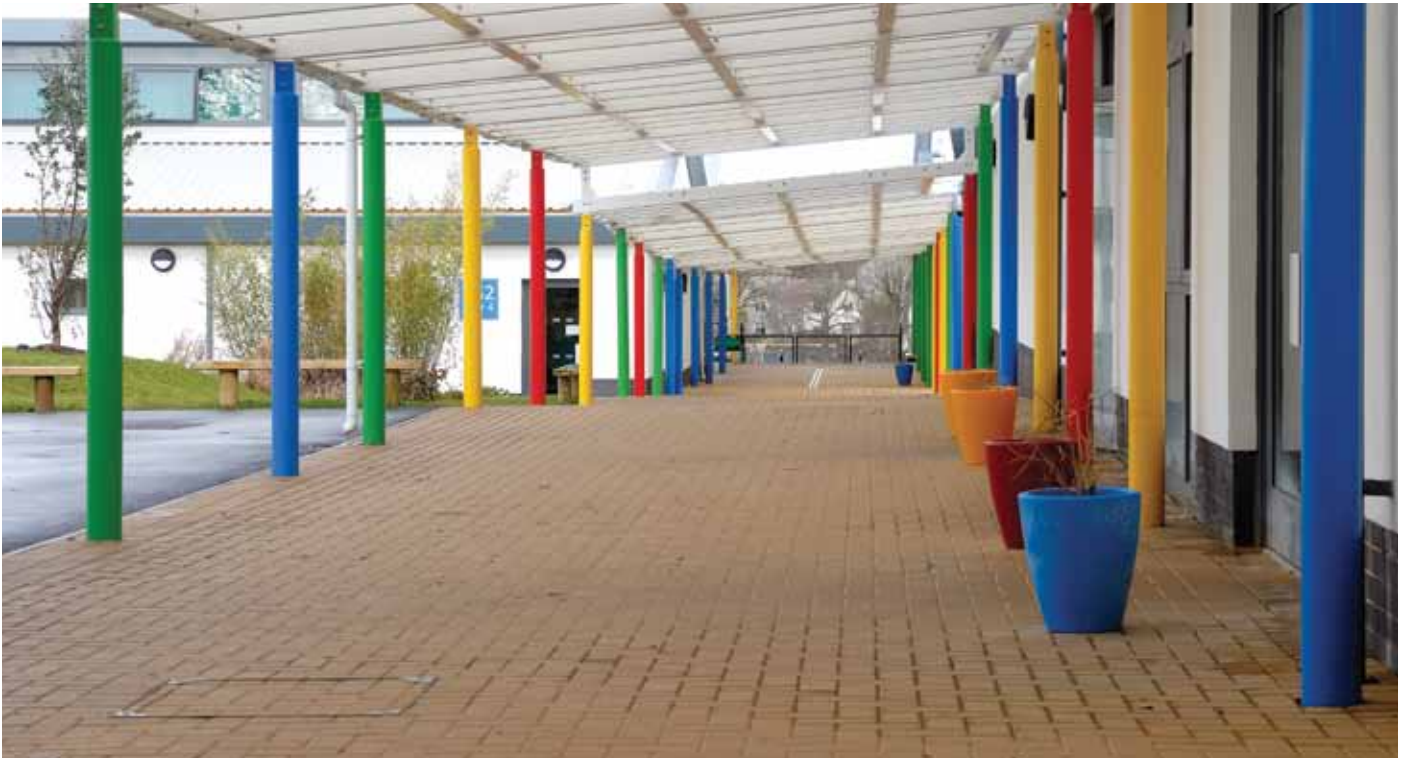
Walkways with support columns in primary colours
