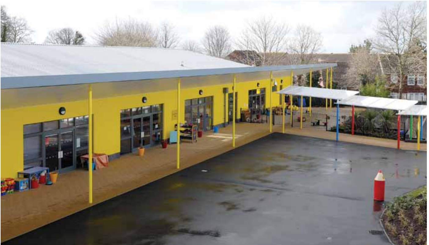
Overview of site showing walkway stepped to suit gradient
