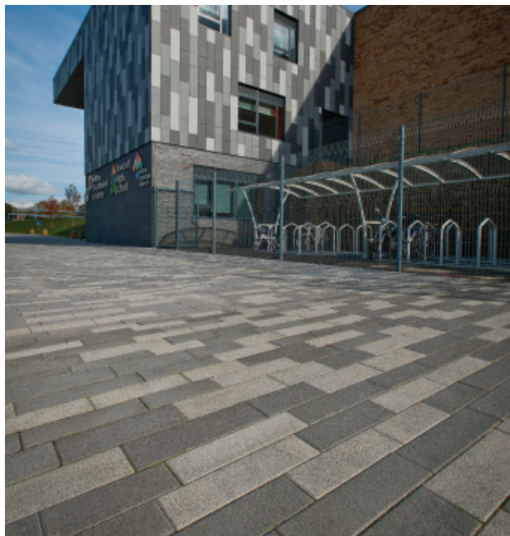
Coordinate with Metrolinia Block Paving
