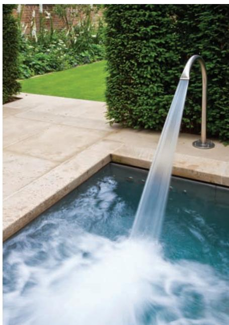
smaller oblong mosaic versions creating a minimalist look. In order to reduce the free board and eliminate the need for skimmers, the York stone coping was cut to form the actual freeboard so that the water appears to be running directly under the coping resulting in an unusual variant of a deck level water flow system.
